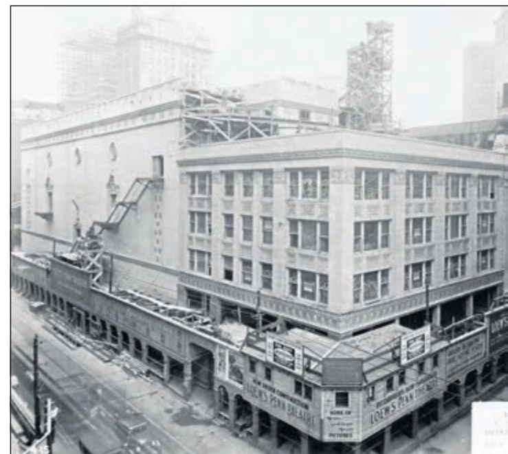
Loew's Penn Theater (now Heinz Hall) construction
