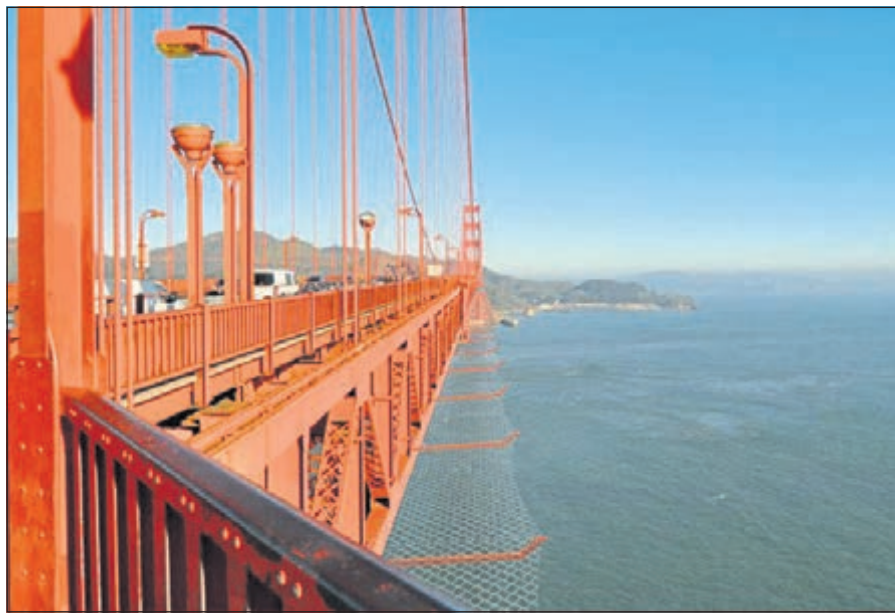
COURTESY OF GOLDEN GATE BRIDGE HIGHWAY AND TRANSPORTATION DISTRICT
